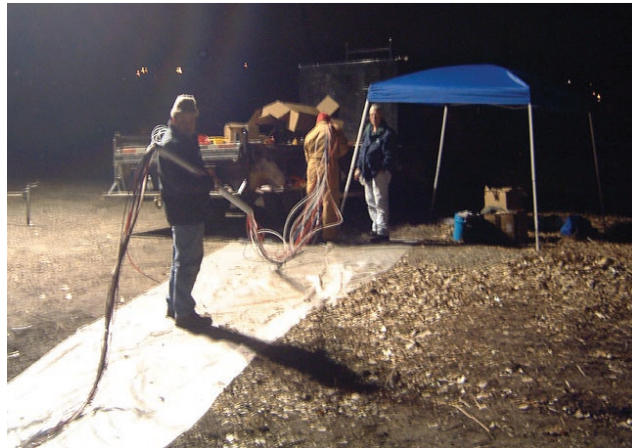
Figure 4-5 Casing Section Being Threaded Over Monitoring Tubing
