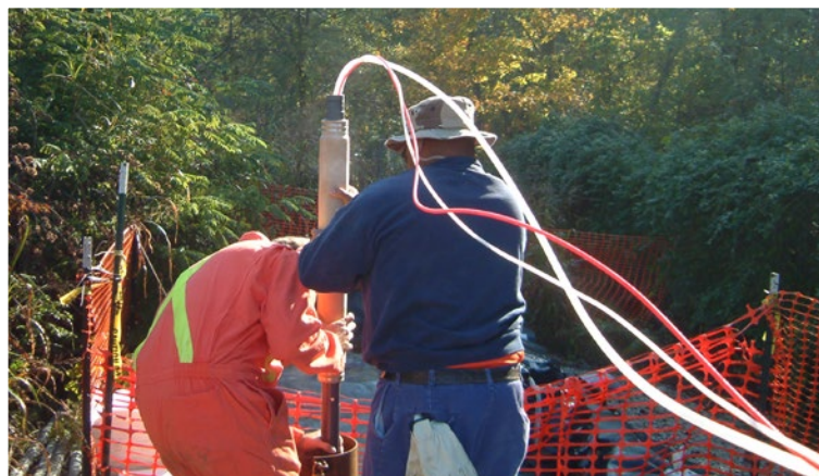
Figure 4-4 Initial Section Being Installed Down-hole
