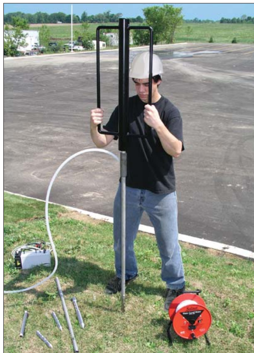
Installing Piezometers with a Manual Slide Hammer
