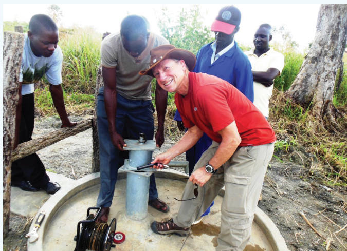
Levellogger Edge being installed in a well near Opit, Uganda.
