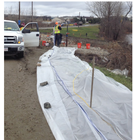
Waterloo Multilevel System installation with double valve pumps and vibrating wire transducers.
