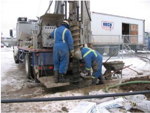
Photo 1: Drilling of the Waterloo Emitters using hollow stem auger in October 2004.
