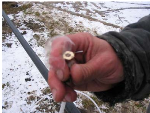
Photo 11: A photo of an air bleed. Air bleed was installed to eliminate any moisture build up and to confirm communication with the oxygen source.
