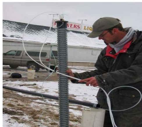
Photo 10: A photo of a connected Waterloo Emitter™ to the two LDPE lines. One LDPE line for incoming oxygen, the second line connected to an air bleed.
