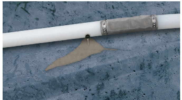
Grout exiting the Grout Plug, below the Port Screen.
